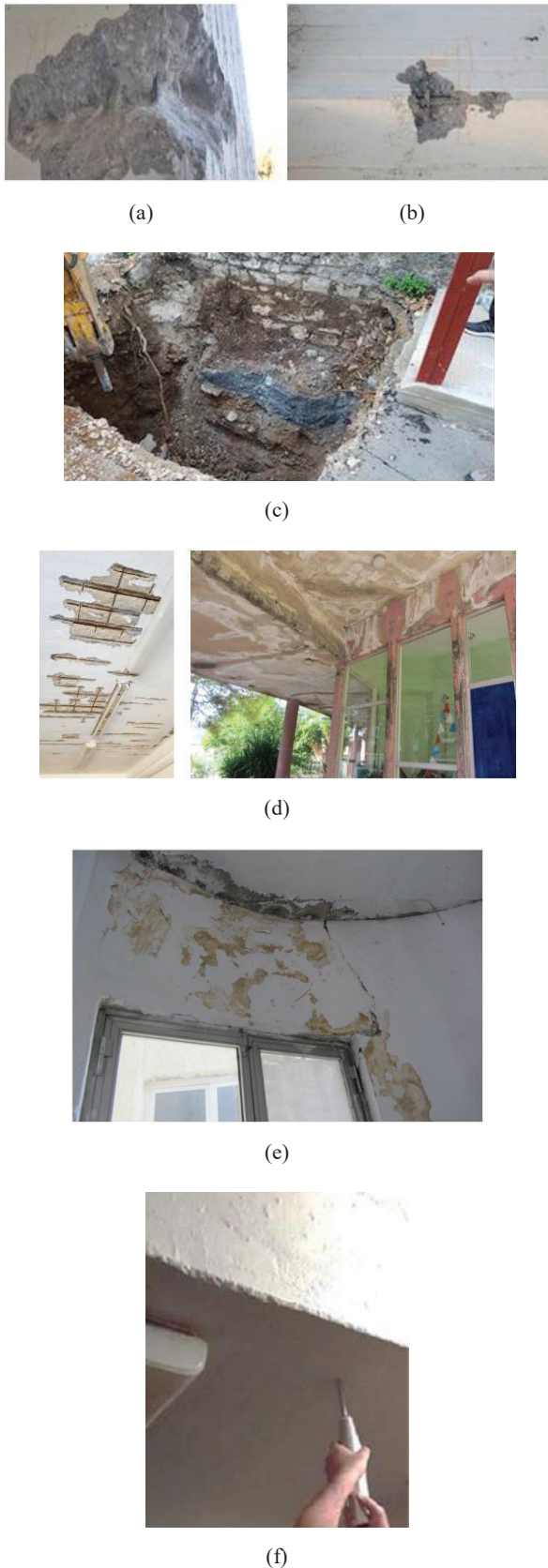
Fig. 3 Disclosure of steel reinforcement materials (a,b), disclosure of the foundation in a column (c), localized damage (d,e), and a non-destructive test (f)
