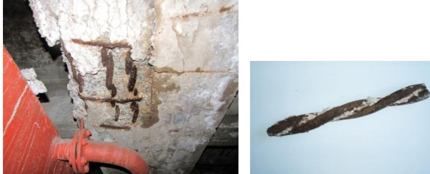
Figure 6: Views of a) a structural member with twin twisted bars and b) a twin twisted bar taken from the field.
