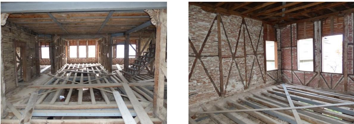
Figure 3: Interior views of the 1st (left) and 2nd (right) floor. The timber framed masonry is clearly visible.
