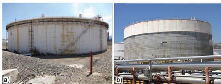
Figure 1: Photographic material for tank T-761 (left) and tank T-776 (right)
