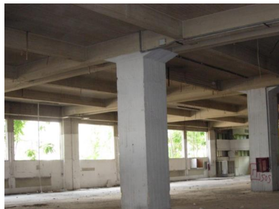
Fig. 2 (a) Exterior and (b) interior views of pre-stressed concrete girders
